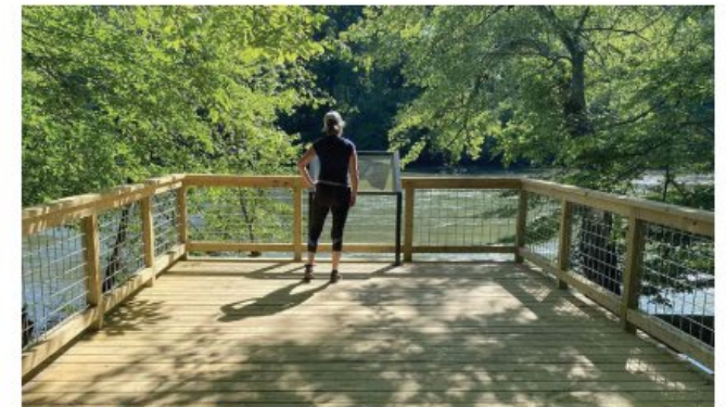
River overlook decking
